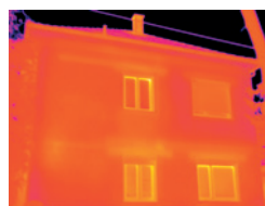
Image thermique sans testo ScaleAssist
