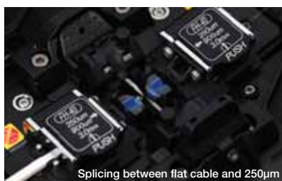
Splicing between flat cable and 250µm
